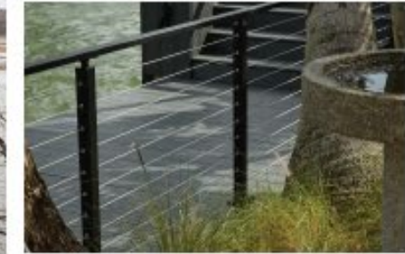
Example Overlook Railing
