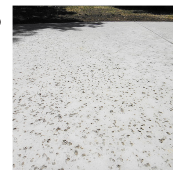
ROCK SALT FINISH CONCRETE
