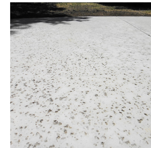
ROCK SALT FINISH CONCRETE
