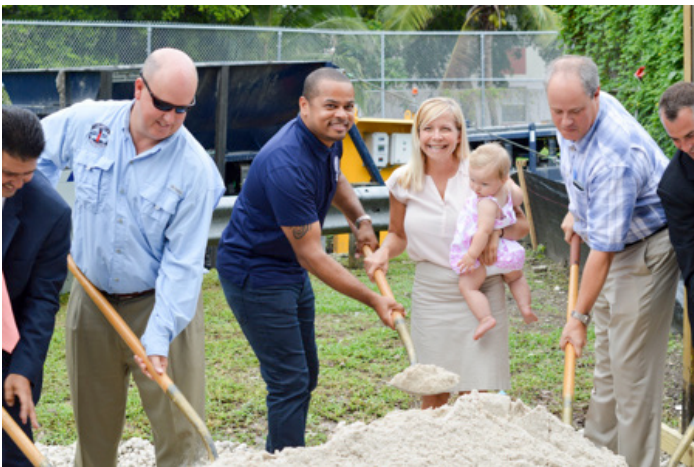
City officials join residents and the Miami River Commission at the Wagner Creek/Seybold Canal Groundbreaking.
