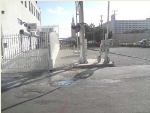
697 N. Miami Avenue (After)
