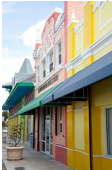
The newly-renovated store fronts along NE 2 Avenue resemble the typical Caribbean style of Haiti. Photo Credit: City of Miami/Jorge R. Perez
